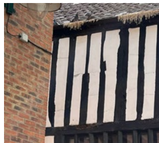
Stained timber in Medieval Buildings with limewash infill panels
