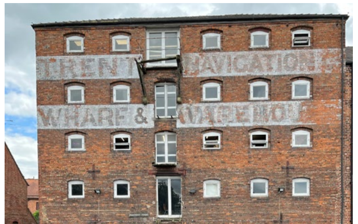
Utilitarian windows, often squarer in proportion: these are found in the industrial buildings and warehouses.
