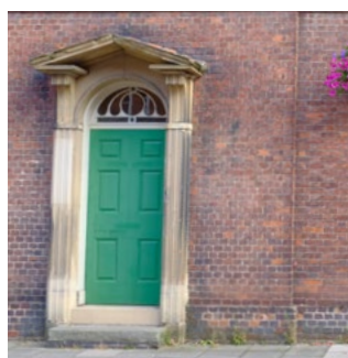
Stone doorcase as a highlight within plain brickwork
