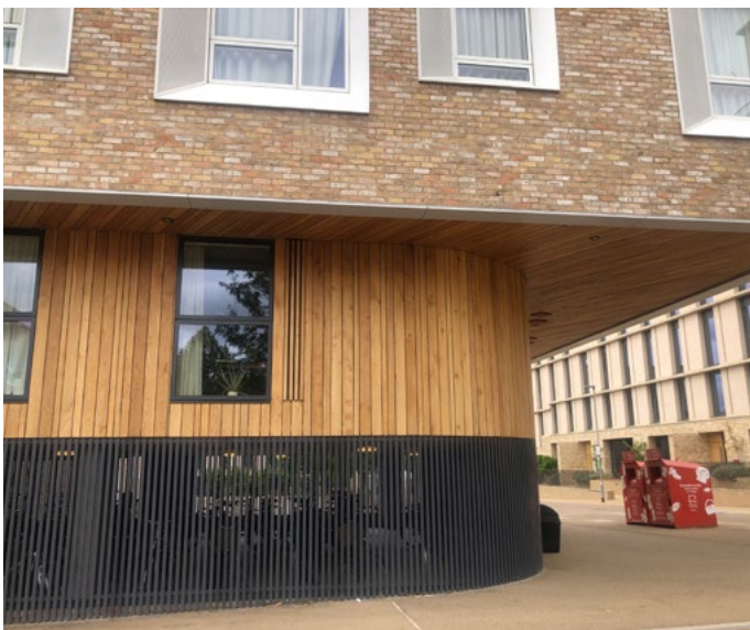
Cambridge cycle parking under apartment block. Photo: Allies and Morrison
