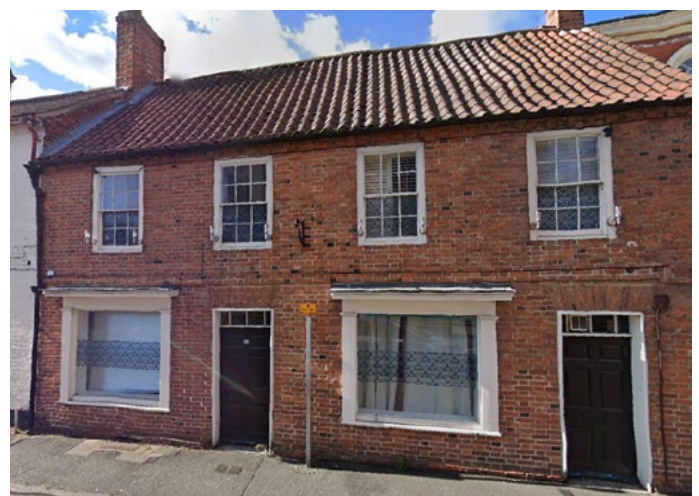
Examples of residential re-use of shop fronts with minimal modification including the use of translucent panels and louvered blinds
