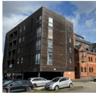
This fully timber clad extension provides contrasting materials in a modern design which clearly distinguishes old from new
