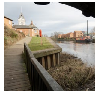
Footpath under Trent Bridge
