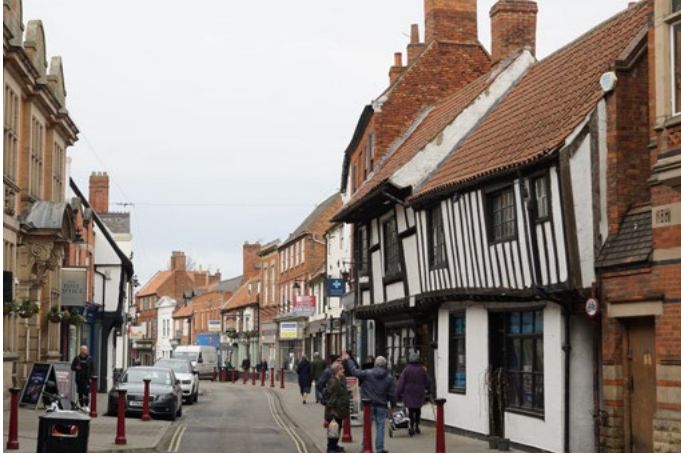
The steeply pitched roof on this medieval building on Carter Gate suggests that it once had a thatched roof
