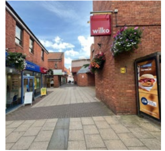
Larger slabs with poor detailing do not reflect the rest of the historic core
