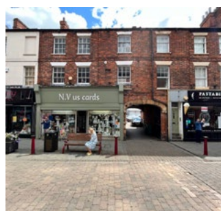
Active shop fronts sit alongside residential doors to upper storeys and restaurants
