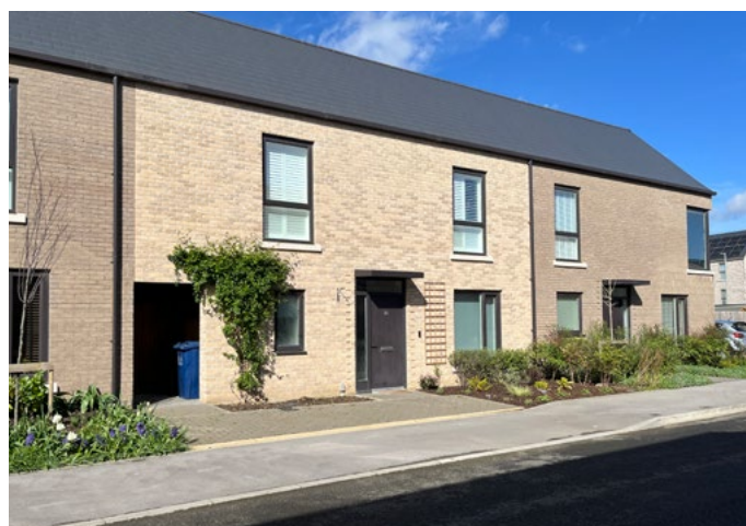
Bin stores integrated into housing keeps footways and front curtilages uncluttered and neat
