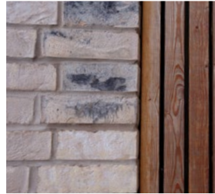
Naturally fired yellow, white, red and black toned brick with natural stained timber
