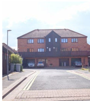
Newer development in North Gate character area incorporates historic materials into road details, such as speed limiting measures and curbs/ gutters
