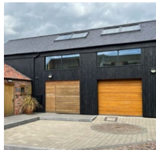
This warehouse-style building located in the historically industrial yards in Mill Gate and Sconce character area successfully utilises a fully dark timber cladding to create a contemporary feel
