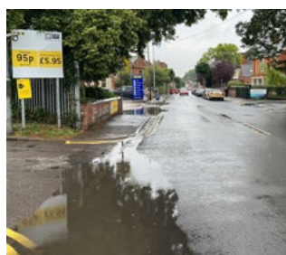
Asphalt is a non-permeable surface and therefore its use should be restricted to carriageways
