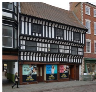
The Governor's House is 'close studded' meaning the wooden structures are close together. The use of this much wood demonstrated the wealth of the owner.
