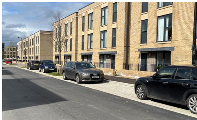
On-street parking with tree planting separating spaces, in Trumpington Meadows, Cambridge
