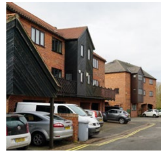
The mix of timber with exposed brick is out of character with Newark and mixed two unconventional materials. However, the timber clad central bay articulates and is in keeping with wharf-style typical in this character area
