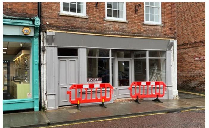
Example of a shop front on Appleton Gate being installed to include clear independent access to the upper floors
