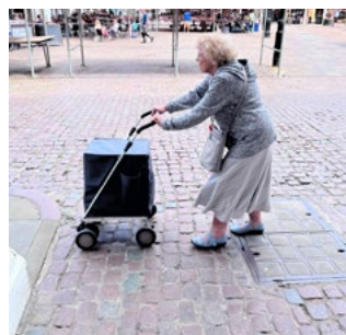
Flattened or shaved cobble setts can help to aid access whilst retaining a historic and heritage character
