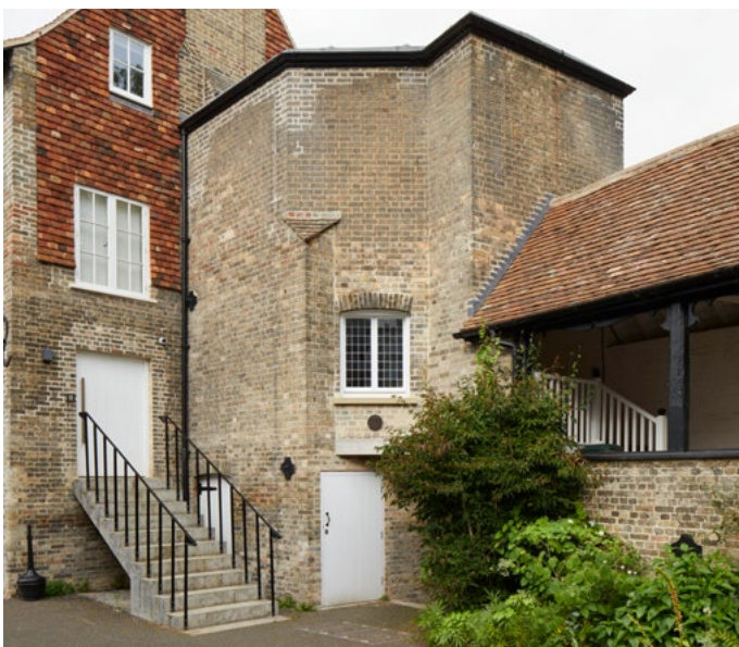
Retrofit to bring building up to a habitable quality at Darwin College Cambridge, including upgrades to doors and windows to improve thermal bridging c. Allies and Morrison
