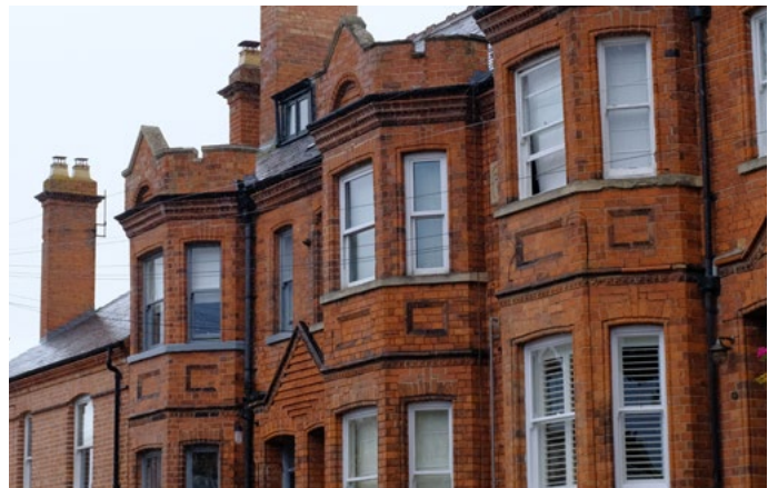
More generously proportioned bays and window groups: these are found in later Victorian and Edwardian buildings
