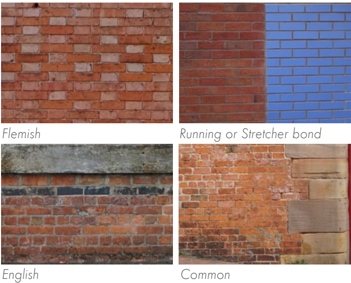
Fig 3 Types of Brick Bonds in seen in Newark
