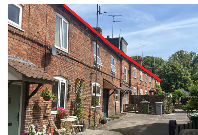
Figure 61: Uniform rooflines example within Southwell
