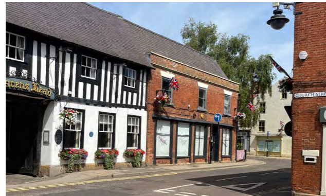
Figure 51: Historical buildings in commercial uses
