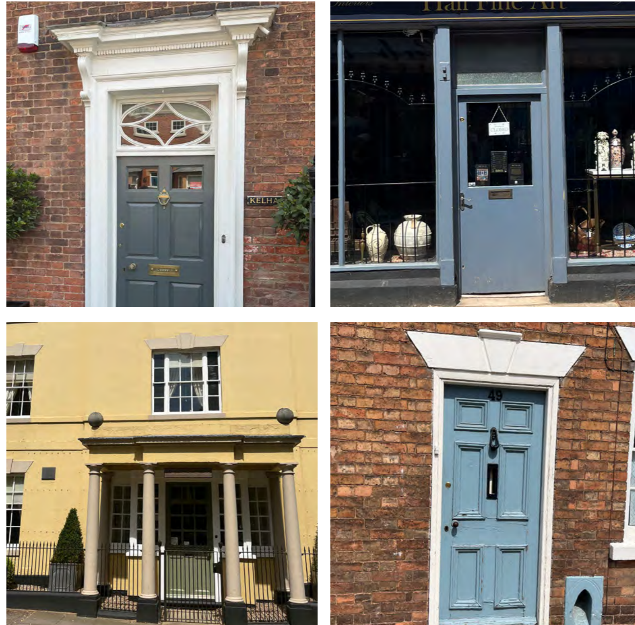
Figure 71: Example of windows and doors
